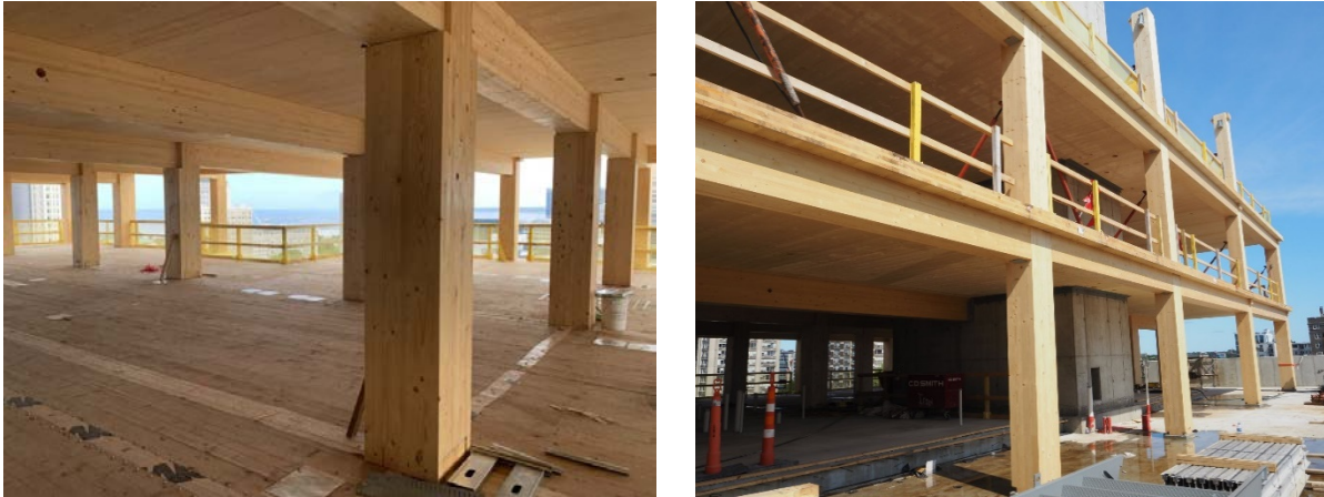
Figure 7 – Building Ascent MKE in the process of assembling structures Source: [11]
