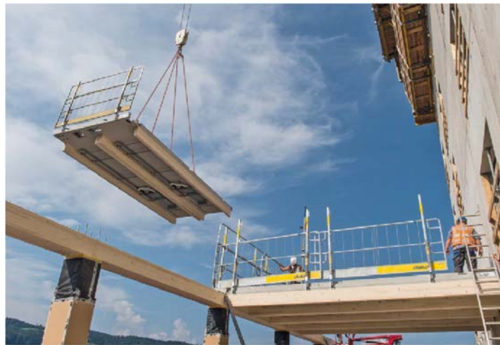
Figure 4 - Installation of a 2.70 m x 6.65 m floor panel Source: [8]
