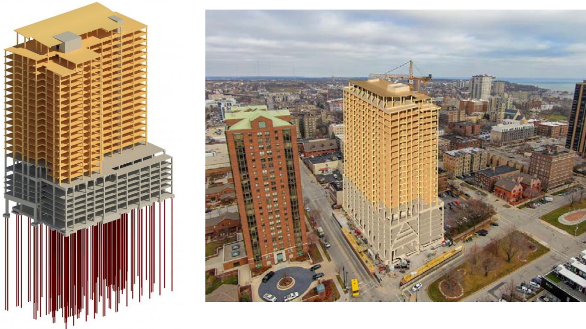
Figure 6 – Ascent MKE, on the left structural model – yellow denotes timber framing, with gray for concrete and red for steel Source: [11]
