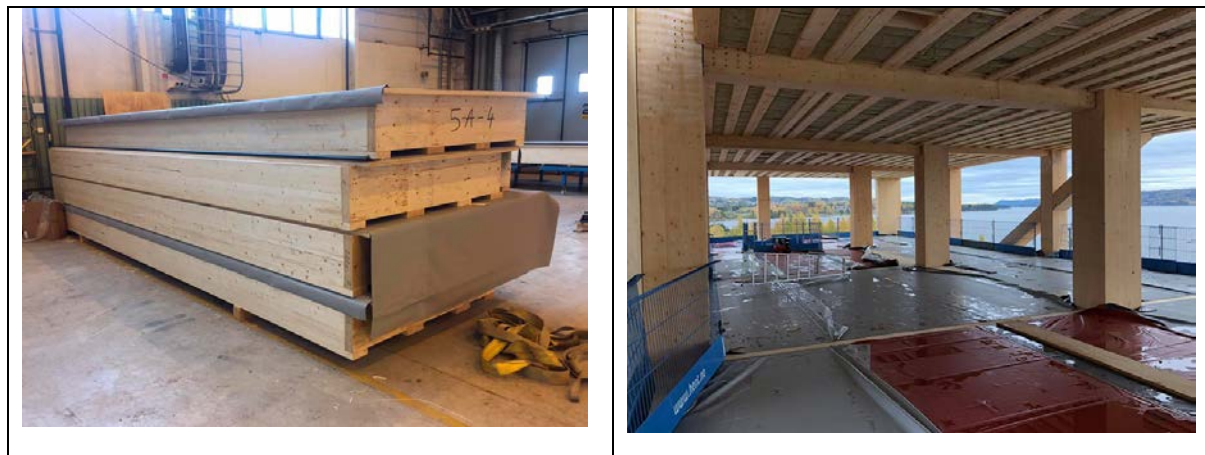
Figure 6 - View of prefabricated sandwich ceiling panels [11]
