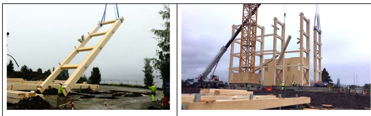
Figure 7 - View of the lifting of 4 storey high structural elements [11]
