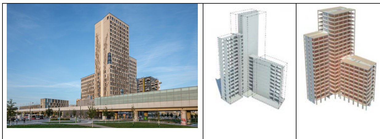
Figure 3 - HoHo Wien - view and illustration of material solution of construction system [7-8]
