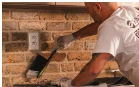
Fig. 13 - Brushing off the excess material
