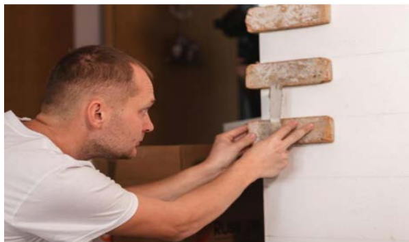
Fig. 10 - Bonding of corner elements
