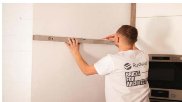
Fig. 8 - Drawing the lines using a spirit level Source: [9]
