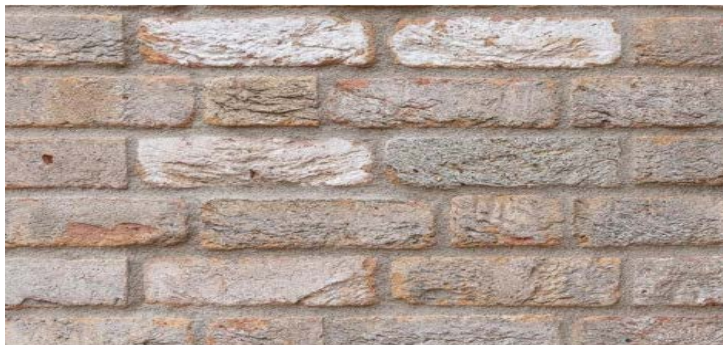
Fig. 14 - Final look of the finished brick cladding
