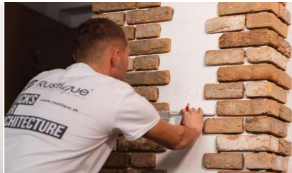
Fig. 11 - Bonding of lining brick slips
