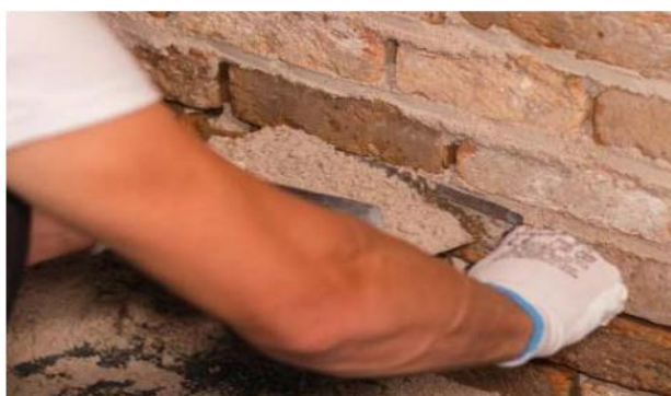
Fig. 12 - Grouting using spatula and trowel
